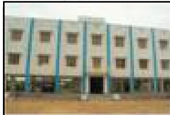
Bhedia Prathamik Vidyalaya Flood Shelter
