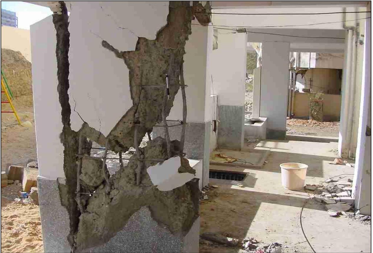
**Figure 6:** 230 mm wide columns in ground storey of RC Frame Buildings: damaged column in Bhuj town during 2001 Bhuj earthquake
