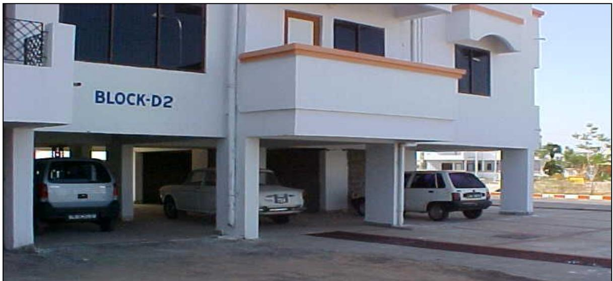
**Figure 5:** RC Frame Buildings with columns in open ground storey of 230mm width
